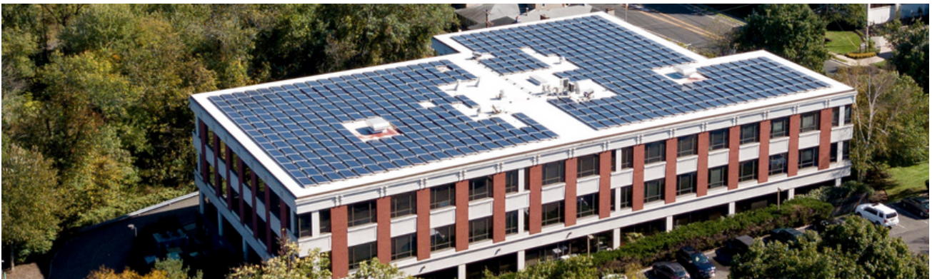
Photo on this page: Aerial view of the Seelaus office building with solar panels.
